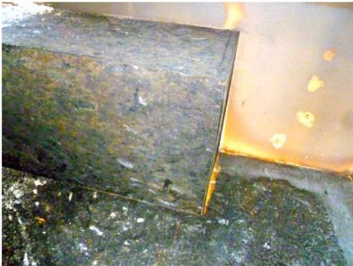
Figure 4 – Minor damage to wood cabinet and gypsum wall board in room of origin
