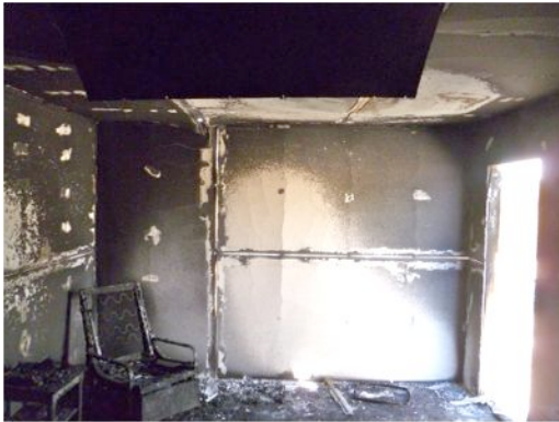
Figure 2 – Area of severe damage coincides with path of inflowing air
