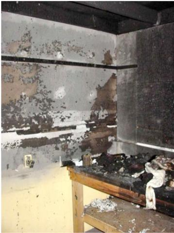
(Fig. 7) Upper layer damage extending down only to base level of fire
