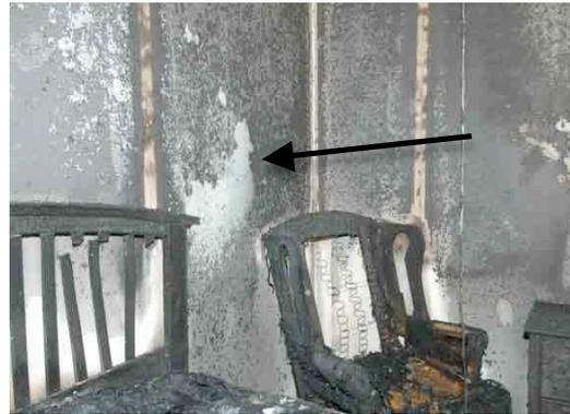
Fig 3 – Closer view of Cell 1 clean burn
